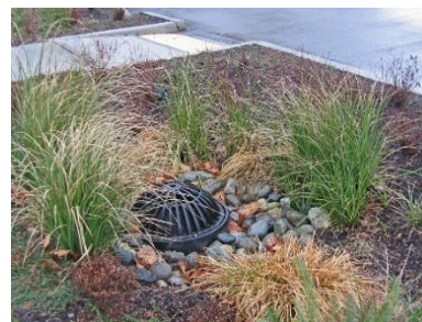
Overflow drain in rain garden swale (photo credit: Brett VA).
