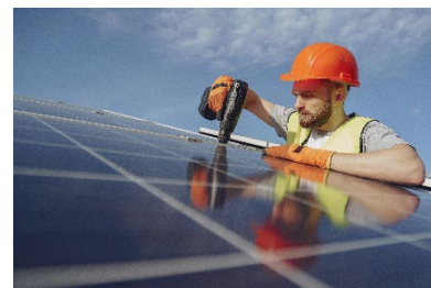
Solar panel installation (photo credit: Gustavo Fring).
