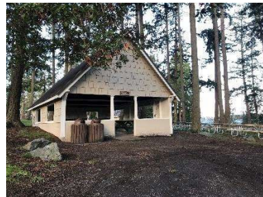
Picnic shelter at Coupeville Town Park.
