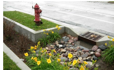
Bioretention swale (photo credit: Aaron Volkening).
