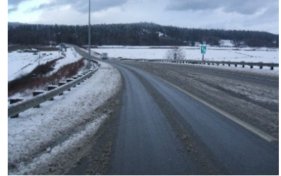
Looking north across Dugalla Bay on SR 20 on Whidbey Island (photo credit: WSDOT).
