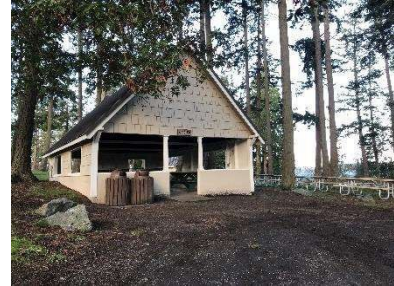
Picnic shelter at Coupeville Town Park.
