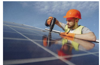
Solar panel installation (photo credit: Gustavo Fring).
