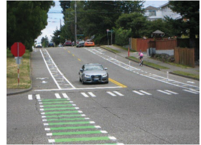
Protected bike lane (photo credit: SDOT).
