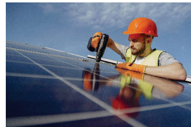
Solar panel installation (photo credit: Gustavo Fring).
