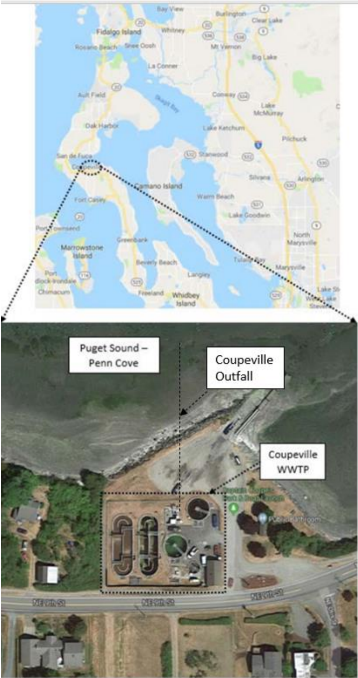
Figure 2-1. Coupeville Wastewater Treatment Plant and Discharge Locations
