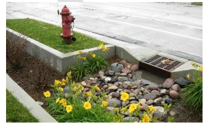
Bioretention swale (photo credit: Aaron Volkening).
