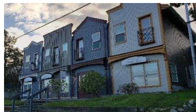
A mixed-use office and lodging building with significant modulation and parking located in the rear.
