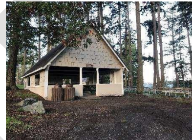
Picnic shelter at Coupeville Town Park.
