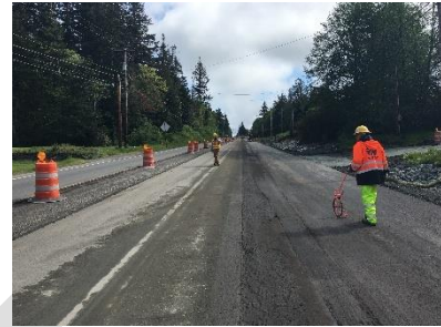
WSDOT contractor crews working on SR 20 (photo credit: WSDOT).
