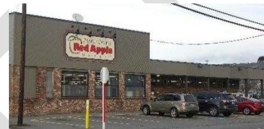
Commercial center in south Coupeville.
