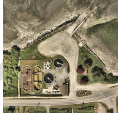
Wastewater treatment plant (photo credit: 2024 ICGeo aerial imagery).
