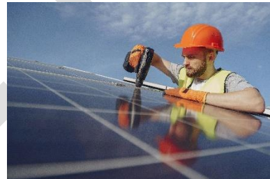
An electrician installing a solar panel (photo credit: Gustavo Fring).
