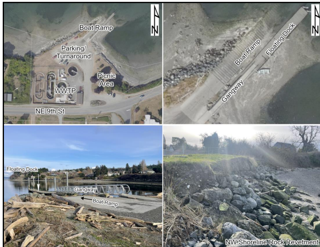
Figure 33. Aerial view and context for Thomas Coupe Park (top left) and boat ramp (top right); site photos of boat ramp (bottom left) and deteriorating rock revetment to west of boat ramp (bottom right).
