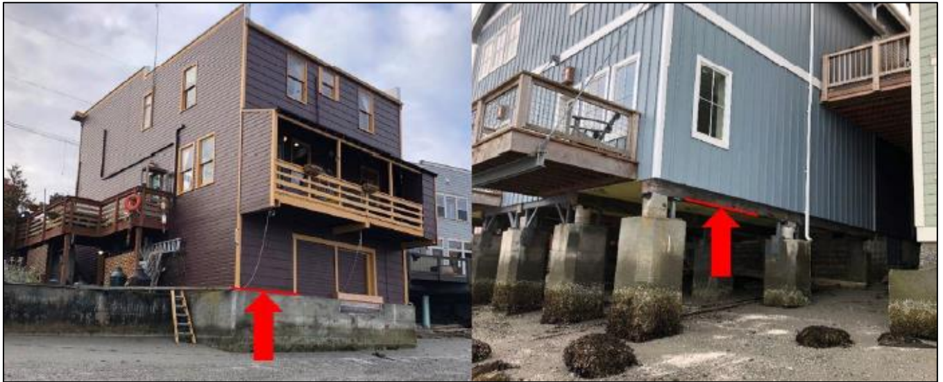
Figure 24. Example showing structures built with concrete foundation (left) and a structure on pilings (right).
