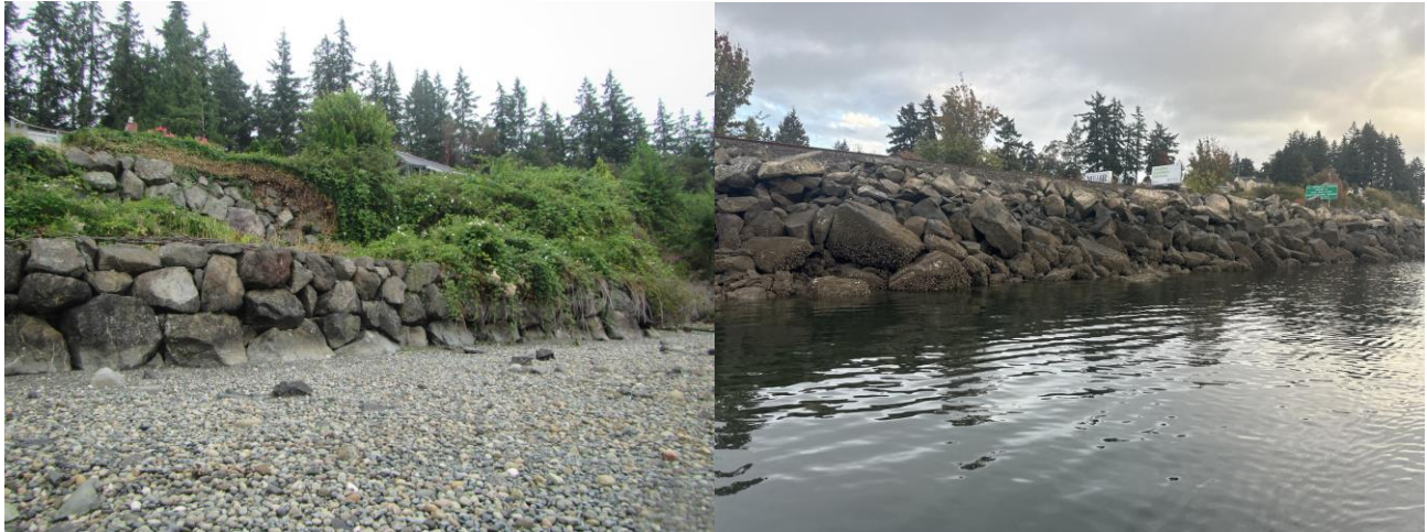
Figure 4. Examples of different forms of rock revetments (Photo Credit: Avery Maverick, 2024)
