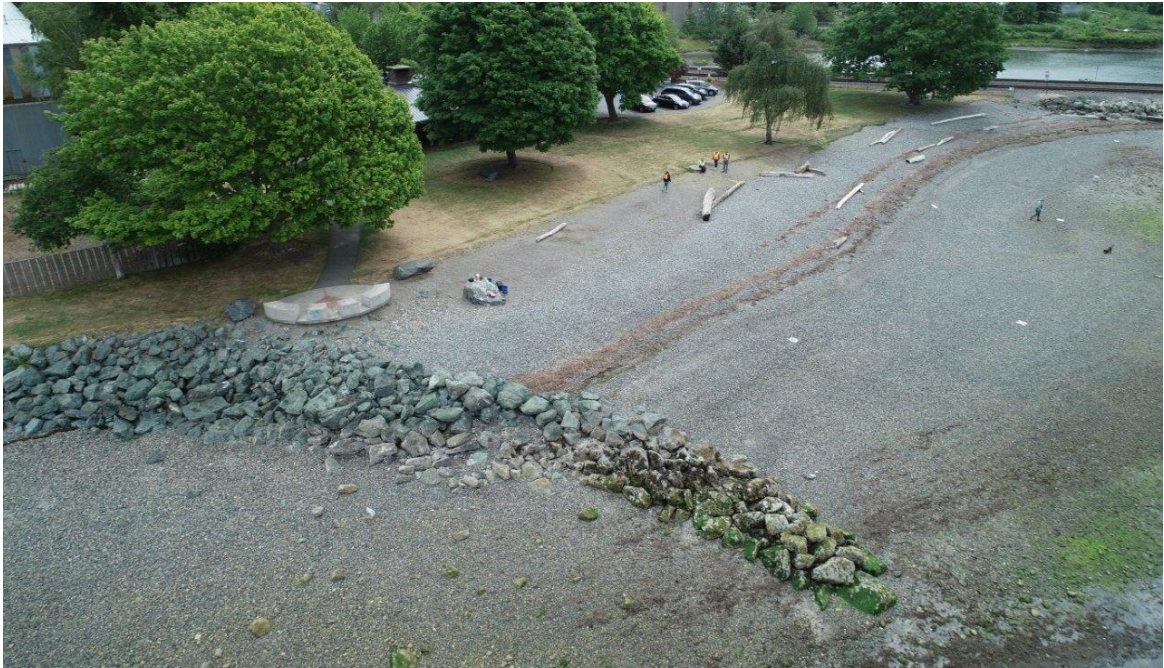
Figure 6. Example of a rock groin at Marine Park in Bellingham, WA (Photo Credit: Adam Tullis, 2021).
