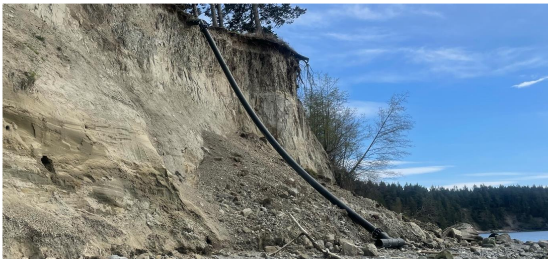
Figure 1. Example of a drainage tightline routed over a bluff (Photo Credit: Avery Maverick, 2021).
