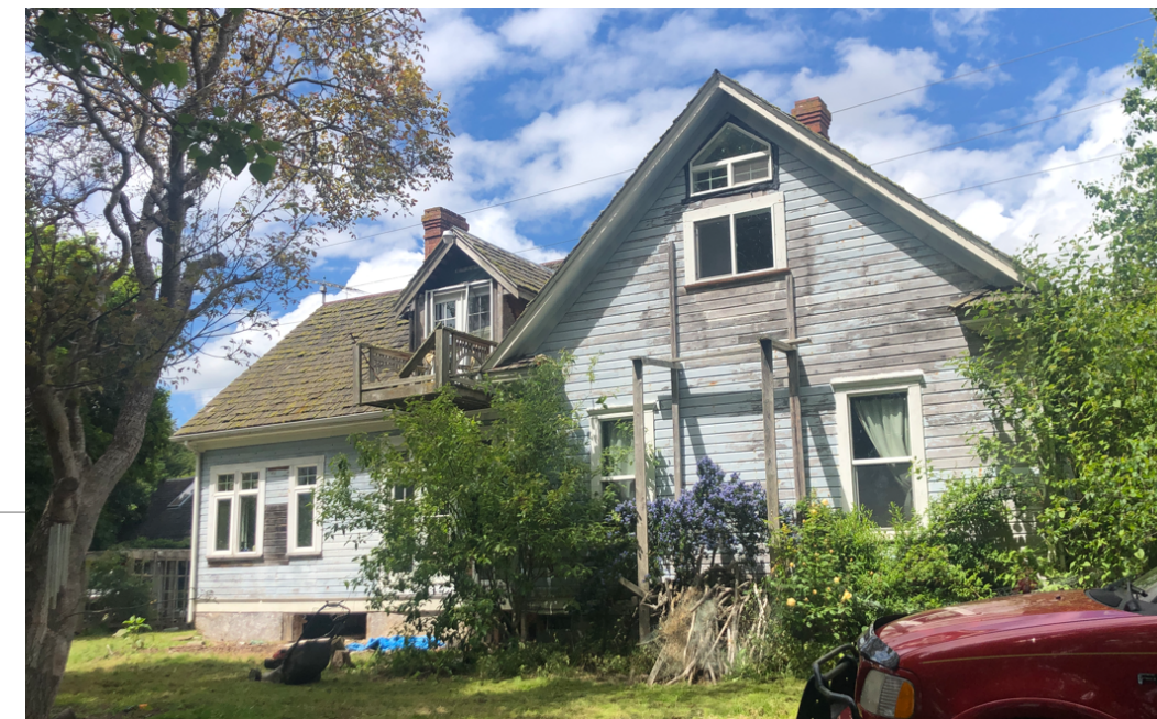
South Elevation Per Property Clean Up
