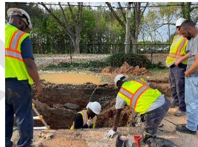
Construction workers inspecting underground utilities (photo credit: Miguel Castillo).
