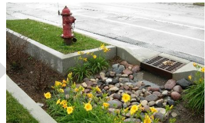
Bioretention swale (photo credit: Aaron Volkening).
