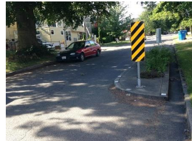
Traffic calming choker (photo credit: Seattle Department of Transportation).
