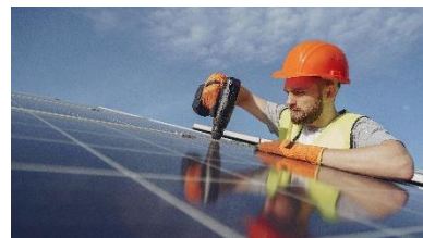
An electrician installing a solar panel (photo credit: Gustavo Fring).
