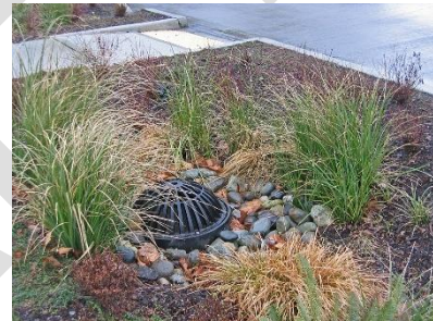
Overflow drain in rain garden swale (photo credit: Brett VA).
