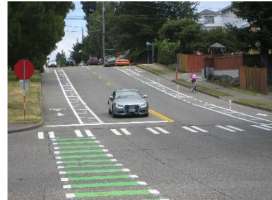
Protected bike lane (photo credit: SDOT).
