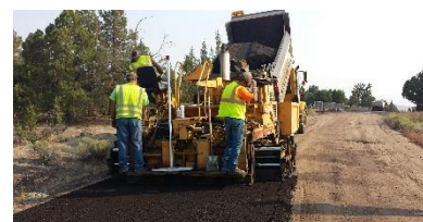
Road maintenance (photo credit: Tom Shamberger).
