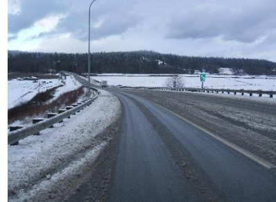
Looking north across Dugualla Bay on SR 20 on Whidbey Island (photo credit: WSDOT).
