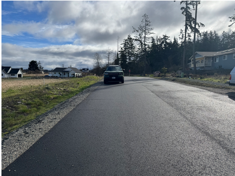
View from the street in front of project Lot 2 / 207 NW 3rd Street looking East.
