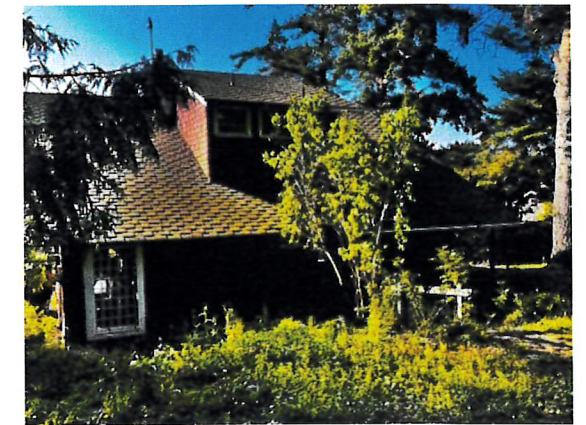
House from N
