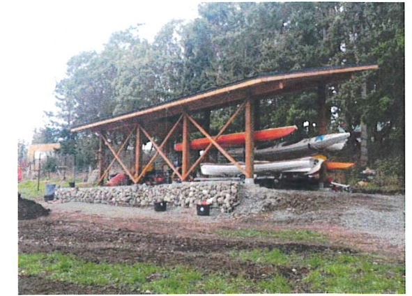
Shed from SE
