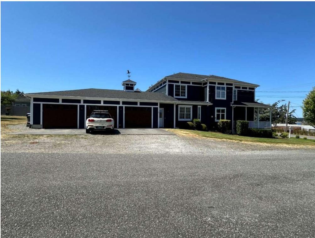
Methodist Parsonage (East Elevation)
