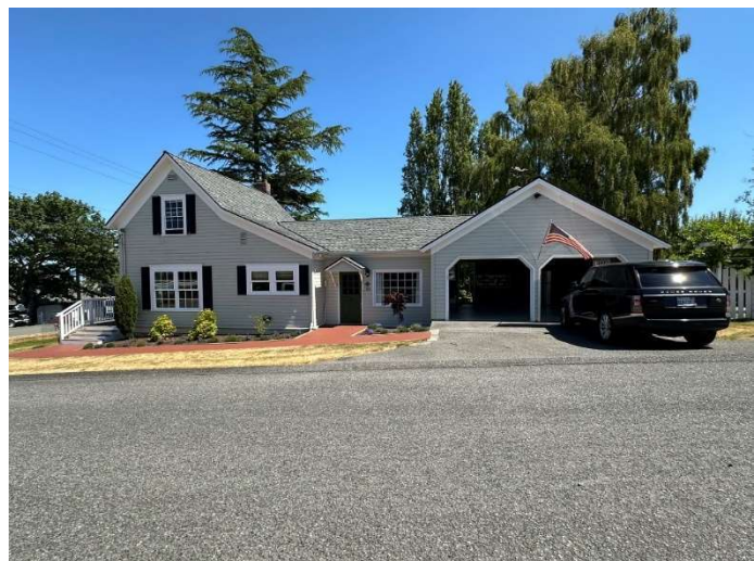
West Elevation (Center Street)
