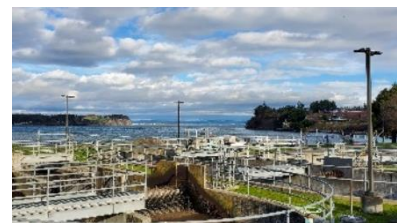
Figure 56 - Coupeville Wastewater Treatment Plant (photo credit: Mary MacPherson)
