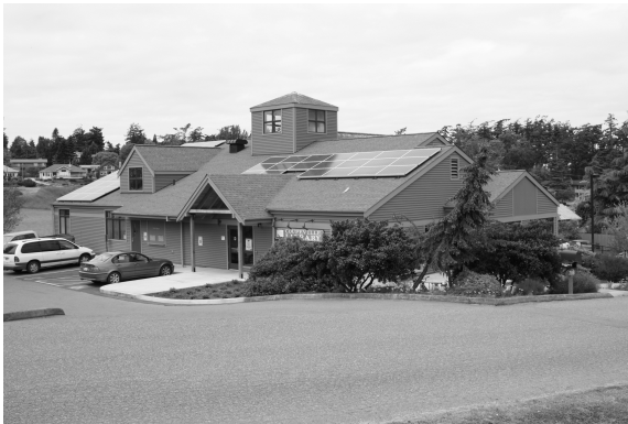
Good Example of compatible installation, below ridgeline, of photovoltaic panels on Coupeville Public Library.
