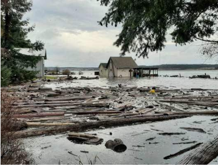
December 27, 2022 – Looking west from northwest corner of parcel – during King tide
