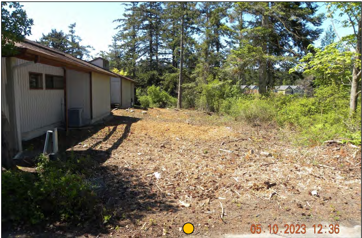
Figure 3: Looking west at generator location.
