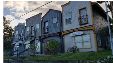
Figure 22 - A mixed-use office and lodging building with significant modulation and parking located in the rear (photo credit: MAKERS)
